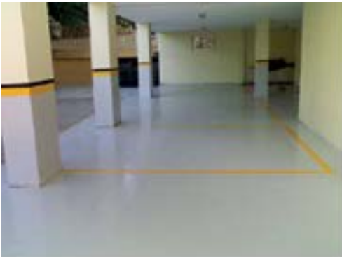
Hasco Chemodur SF - Garage Private Residence
